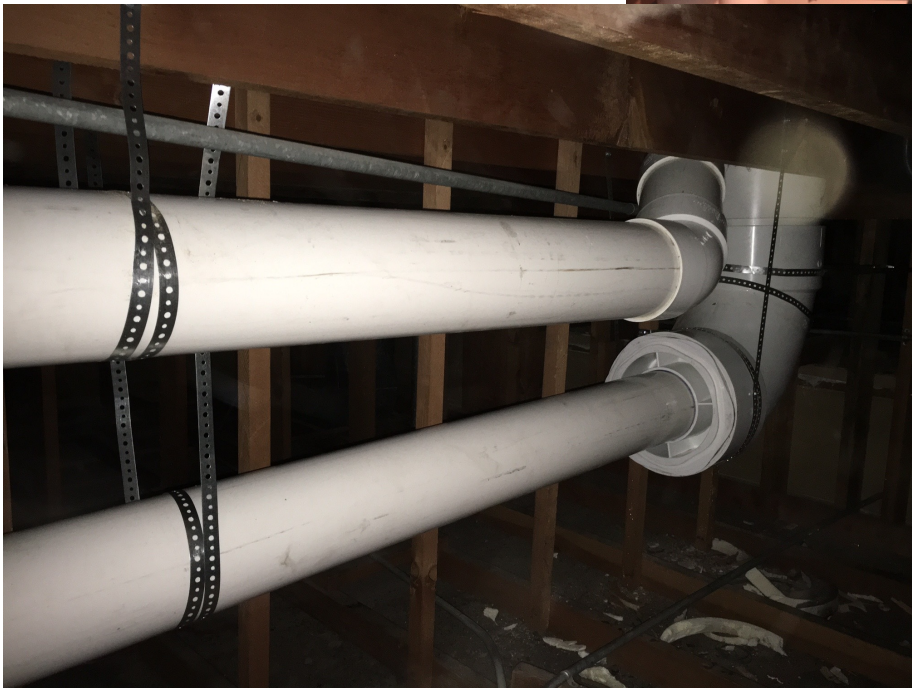
6 inch vent piping converging to 12 inch vent piping through the roof and connecting to the fan.
