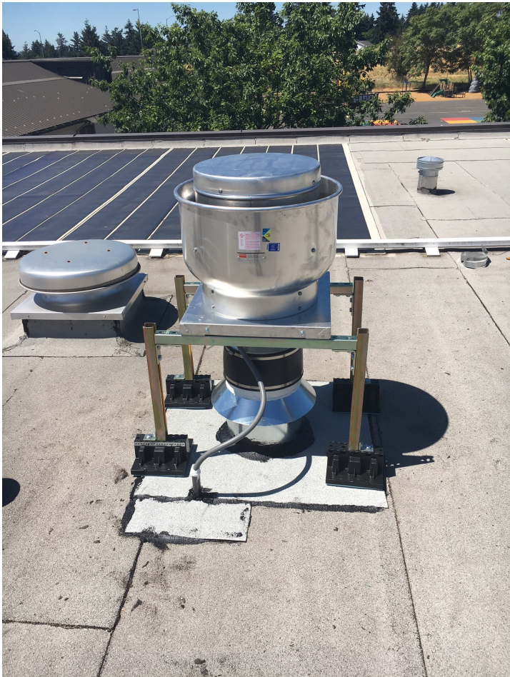
Southern mitigation fan
