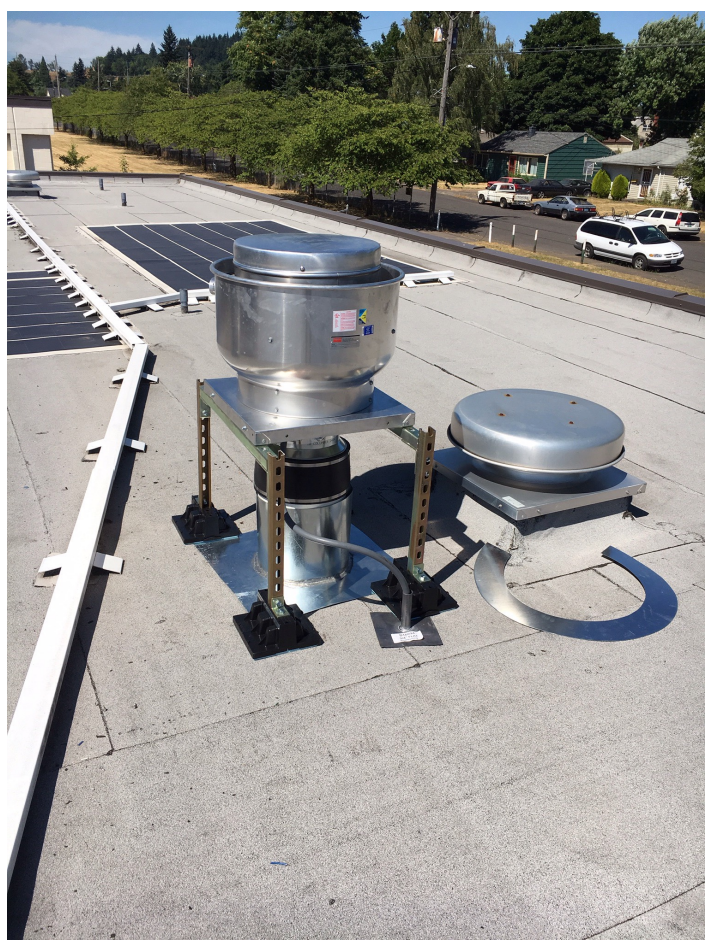
Northern mitigation fan
